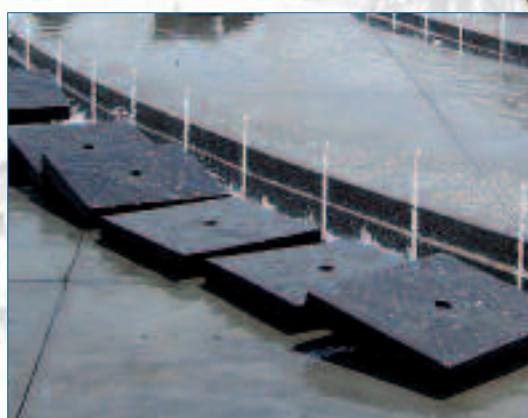
Example of holes drilled directly into the stone slabs. this solution does not allow passing of the beam of the lights.
