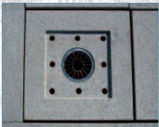
Example of a small size grate. As it limits the beam of light it is suitable for jets of limited height.
