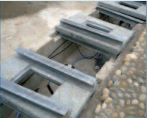
The stone slabs are supported by a steel structure, arranged so as not to interfere with the equipments.
